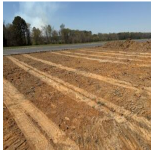
Proof roll conducted West side of storm drain pipe
