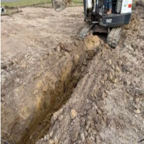
Duct bank trench
