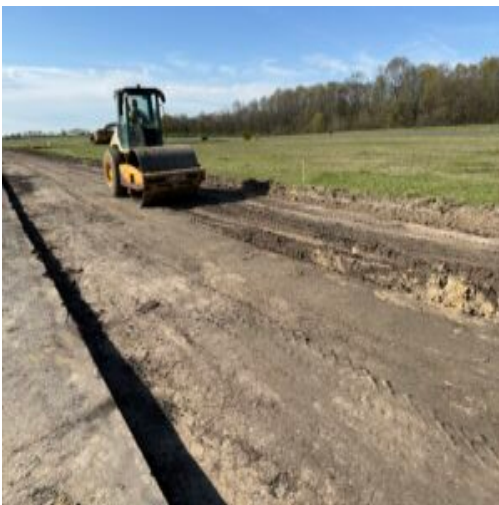
compacting subgrade on A3 & A4 connector
