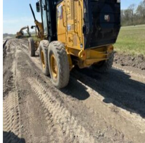
Proof roll conducted between A3 & A4 connector with a motorgrader.
