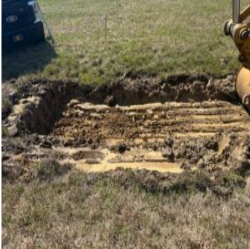
Excavation of Storm pipe location at taxiway A4
