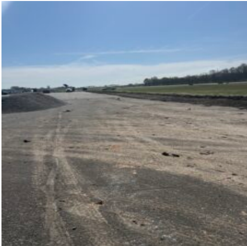
12 inches of excavation for connector between A3 & A4
