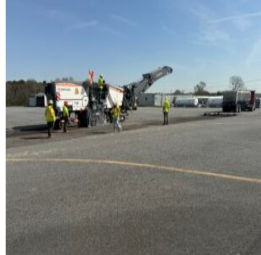
Milling of A3 asphalt
