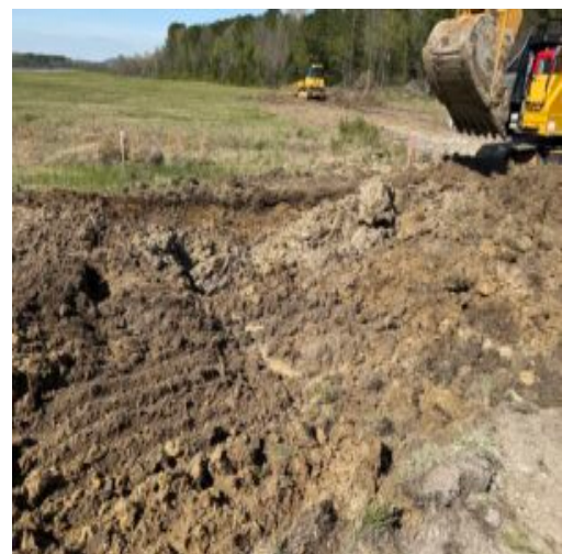
Organic material found as excavating commenced at A4 and connector.
