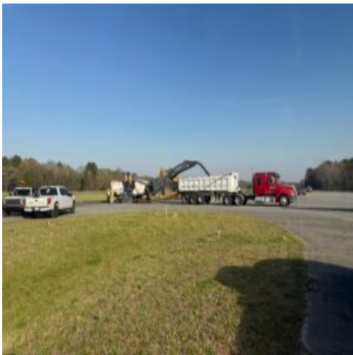
Milling of A3 asphalt
