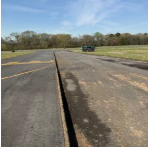
North side of A3 taxiway Milled
