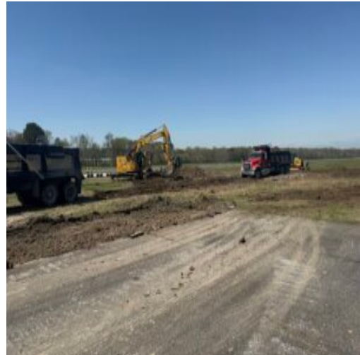
Excavation of future A4 Taxiway
