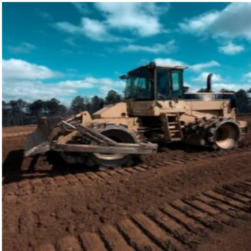
Compacting with 815 equipment
