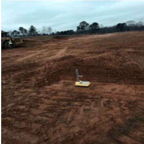
Density tests using Nuclear gauge
