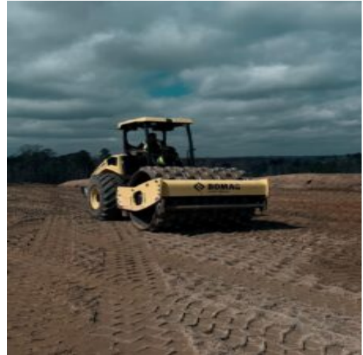
Compacting with sheep foot roller
