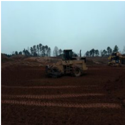
Compacting with 815 equipment
