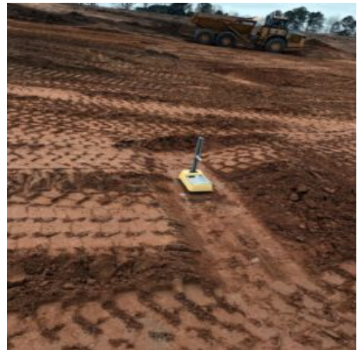
Density tests using Nuclear gauge
