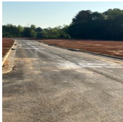
Areas of roadways that was saw cut
