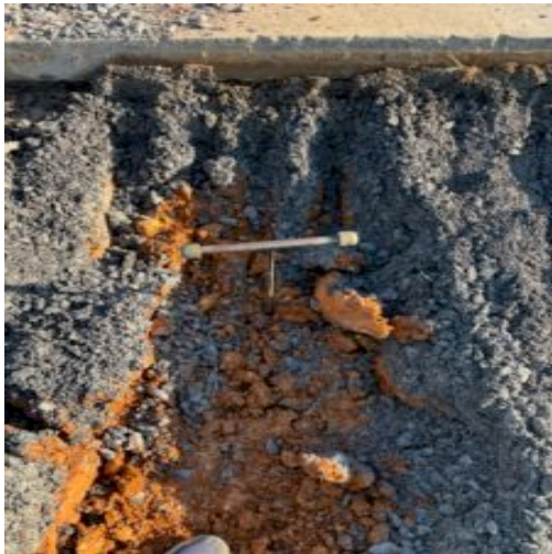
Probing backfill soils
