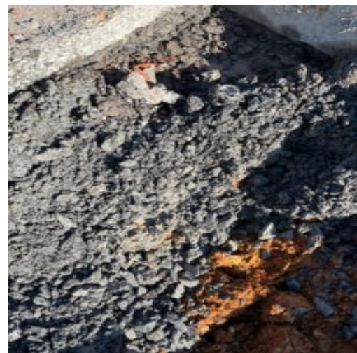
Saturated base stone
