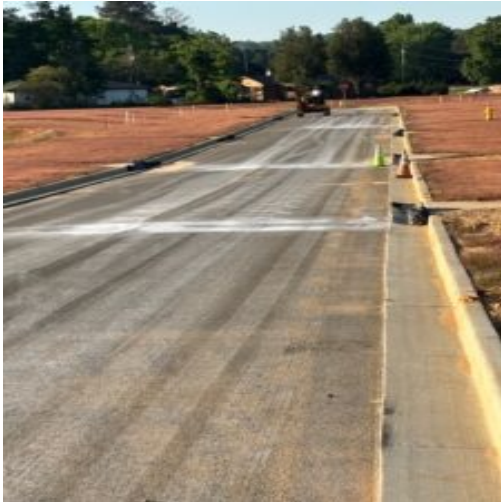
Areas of roadways that was saw cut
