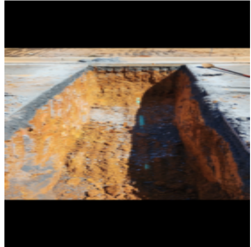
First hole undercut
