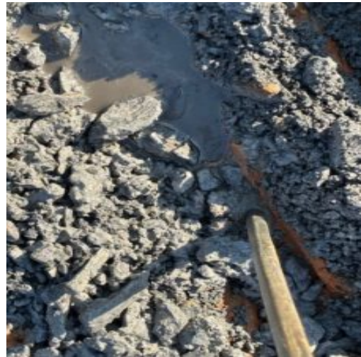
Saturated base stone
