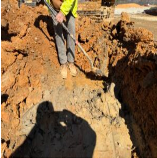
Wet area from water line
