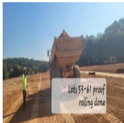
Picture depicting lots 32-35 under backfilling stage Picture showing lots 53-61 proof rolled and passed
