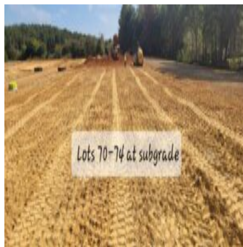
Picture depicting lots 70-74 at subgrade and proof rolled
