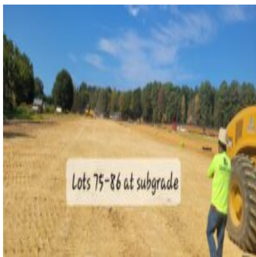
Picture depicting lots 75-86 at subgrade and proof rolled
