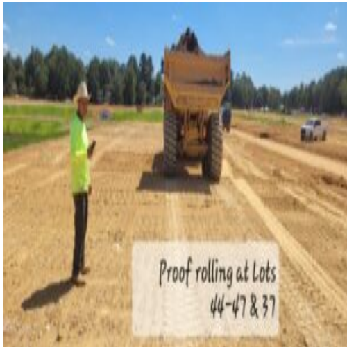
Rechecking of failed compaction of lots being proof rolled
