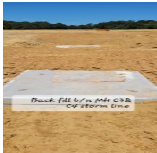
Storm line cutting a road backfilled and compacted
