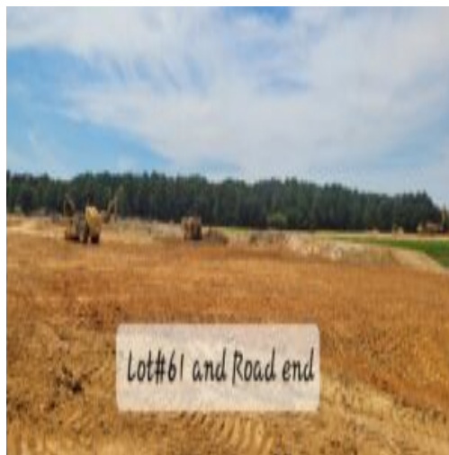
Picttture depicting the road and Lot#61 under backfilling
