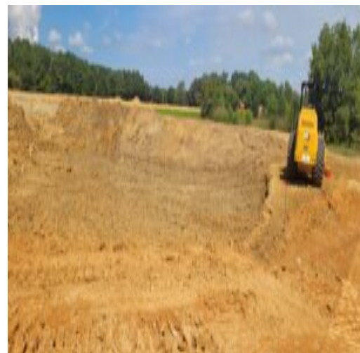
The above excavated surface after bridging and rolling
