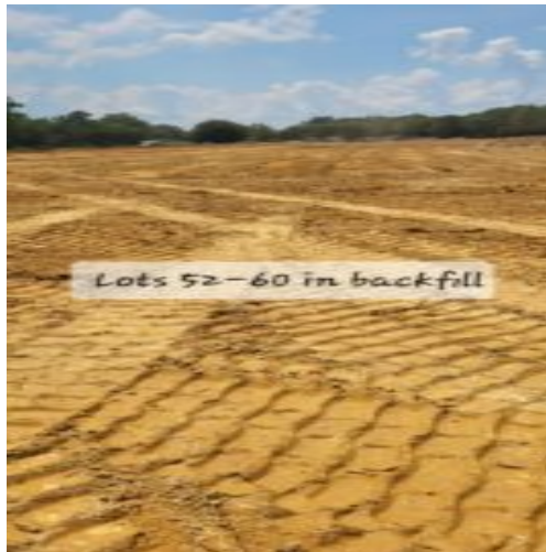
Picture depicting lots 52-60/under backfill activity and 3-6' to subgrade
