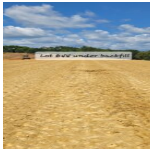
Picture showing lot#44 under backfilling
