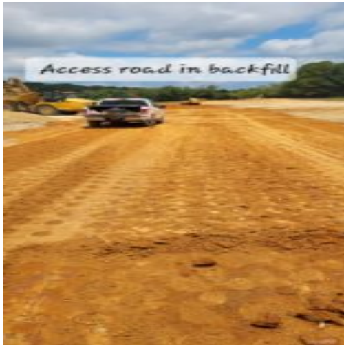
Access road in backfilling at -1' for subgrade
