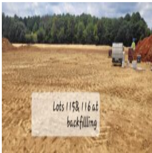
Picture depicting two lots at backfilling and -1' to subgrade
