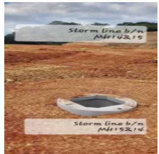
Storm line backfill b/n manholes 14&15
