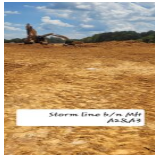
Picture showing storm line b/n Man holes A2 & A3 backfilled and compacted
