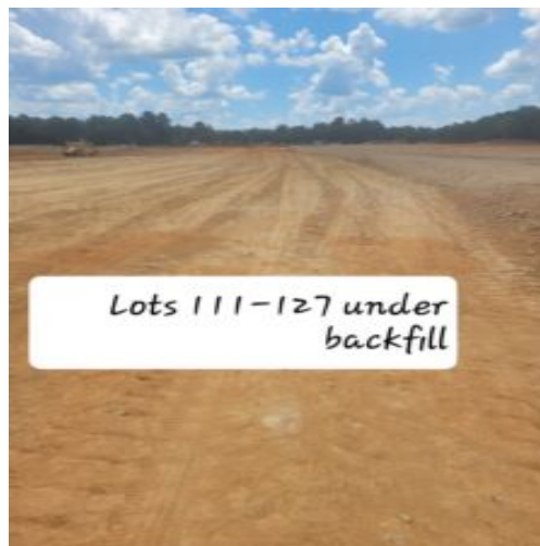
Picture showing lots 111-127 under back filling
