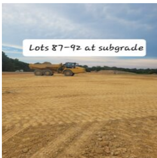
Picture depicting lots 87-92 at subgrade
