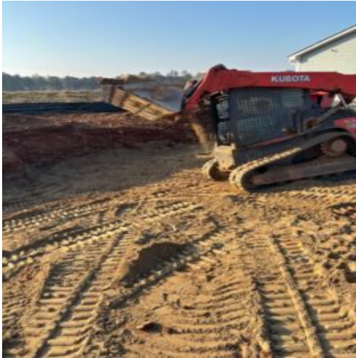
Compacting in place mixed materials using skid loader
