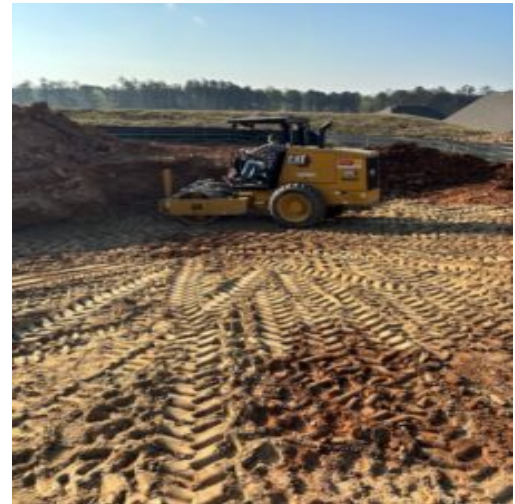
Compacting in place mixed materials using small vibratory sheet foot roller
