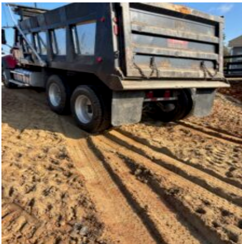
Additional compacting efforts using a tandem dump truck
