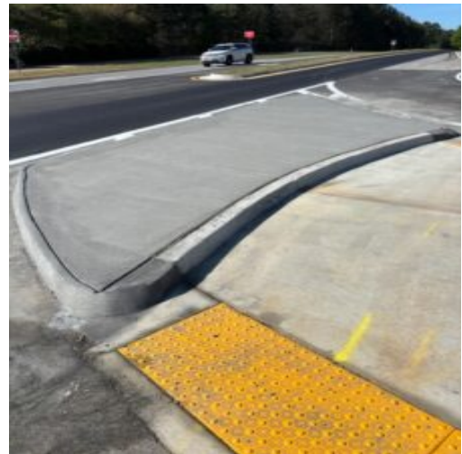
Poured in place pork chop at Seven Hills Boulevard
