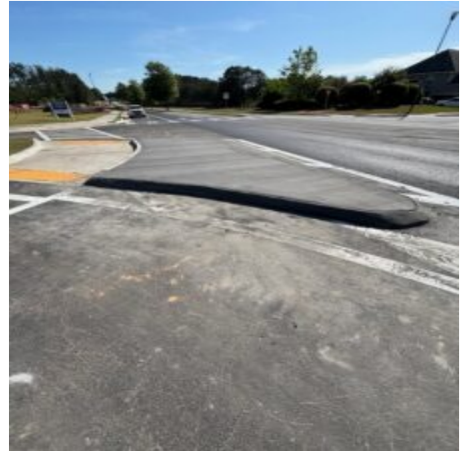
Poured in place pork chop at Seven Hills Boulevard
