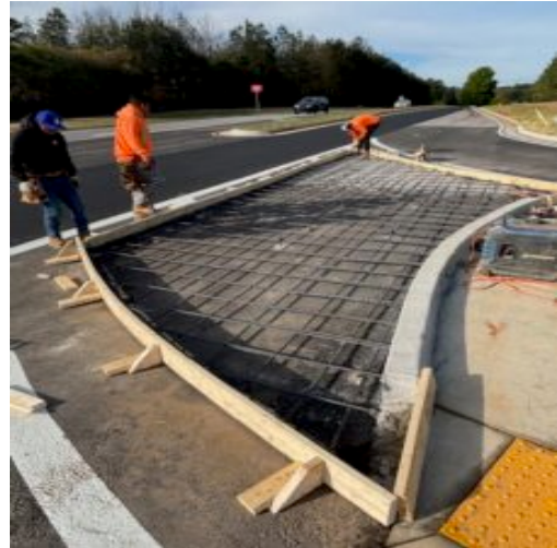
Form work being installed for type 7 curbing.
