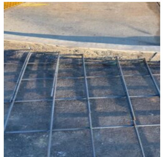
Reinforcing steel observed with deficiencies noted, radius not installed, mat steel not supported by dowels, and forming for curbing not completed.
