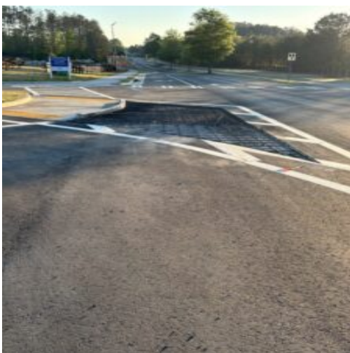
Reinforcing steel observed with deficiencies noted, radius not installed, mat steel not supported by dowels, and forming for curbing not completed.
