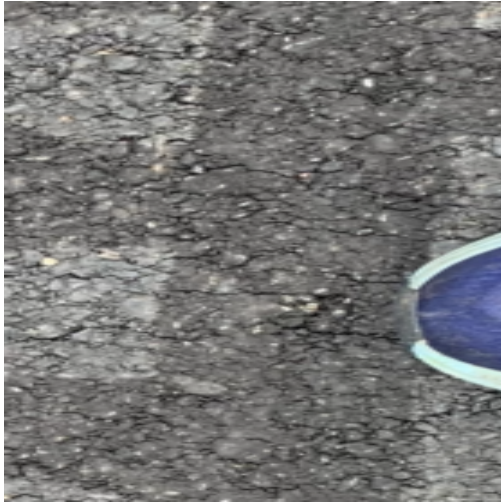
Showing surface cracking at decel lane east side
