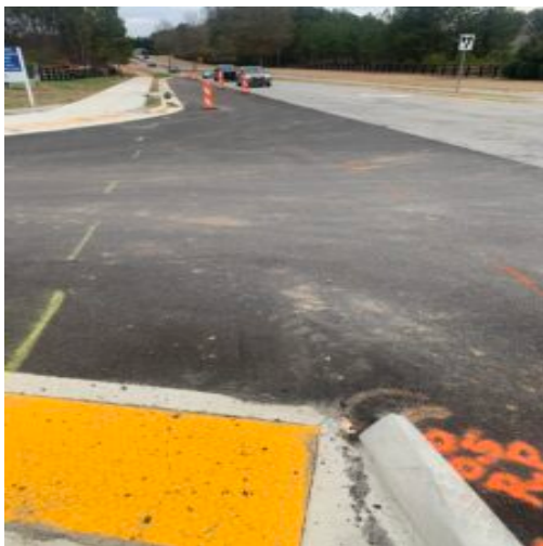
Area to be milled 9.5 "and replaced with class B concrete and topping mix
