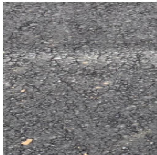
showing surface cracking at east side decel lane
