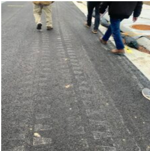
East side decel lane showing topping mix
