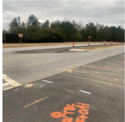
Showing west side decel lane to be milled and replace topping
