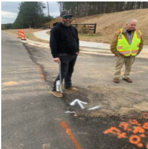
Showing surface cracking at decel lane east side
