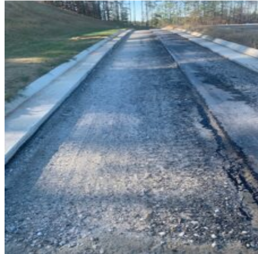
Milled repaired area at exit lane showing depths of 7.25 to 7.50" outside edge and 4" inside
