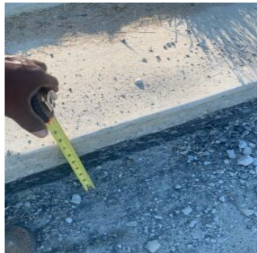
Milled repaired area at exit lane showing depths of 7.25 to 7.50" outside edge and 4" inside
