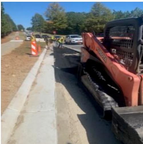
25mm paving at east side decel.lane
