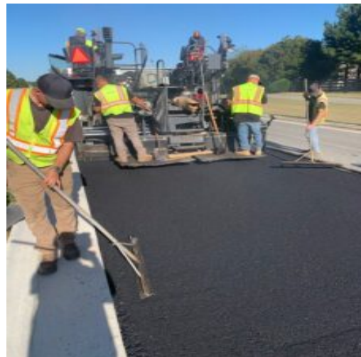
25mm paving at west side decel.lane
