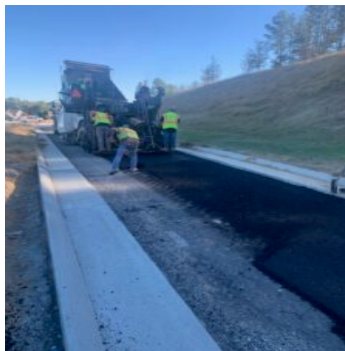
Paving 25mm at repair exit lane
