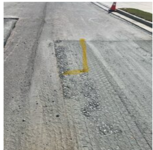
Small isolated area for repair
