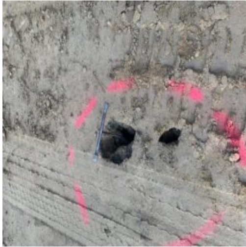
Drill rock holes with voids, recommended to fill with #89 stone
