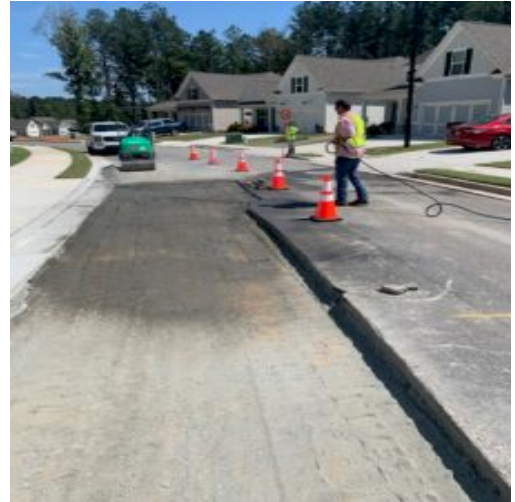
Wetting and compacting subbase stone
