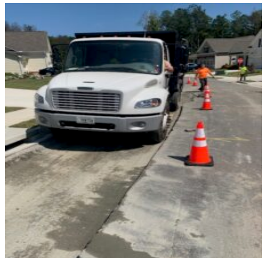
Practice test roll with small truck
