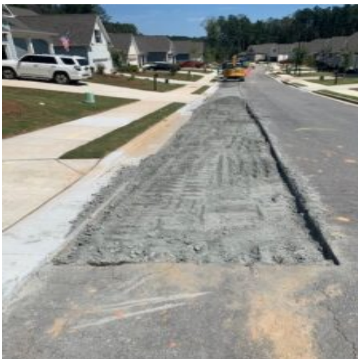
Replacing subbase stone
