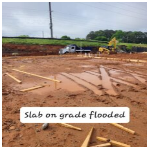
Picture depicting flooded slab on grade
