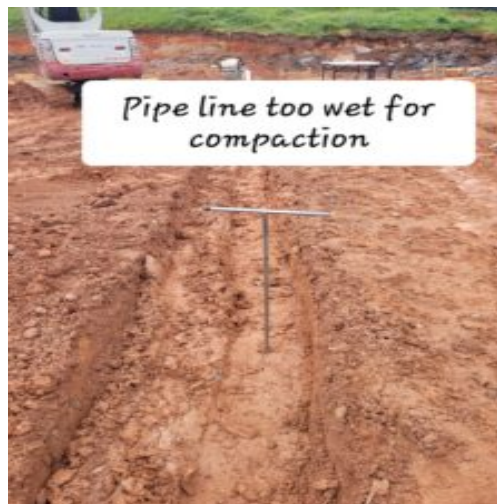
Picture showing too wet surface for compaction.
