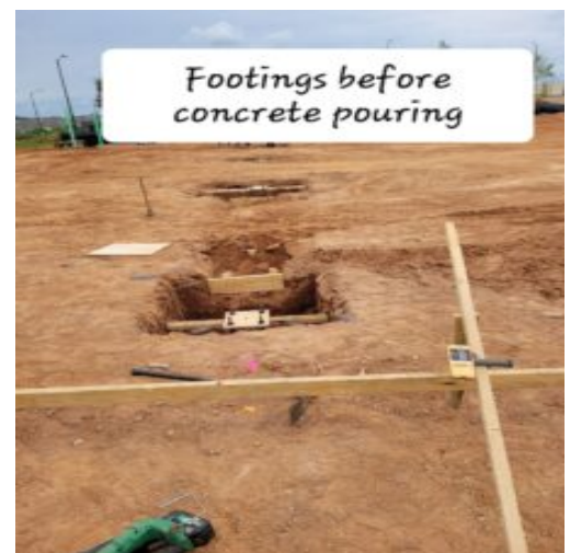
Spread footings before concrete pouring
