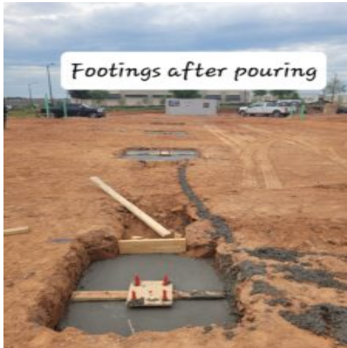
Picture depicting concrete poured footings
