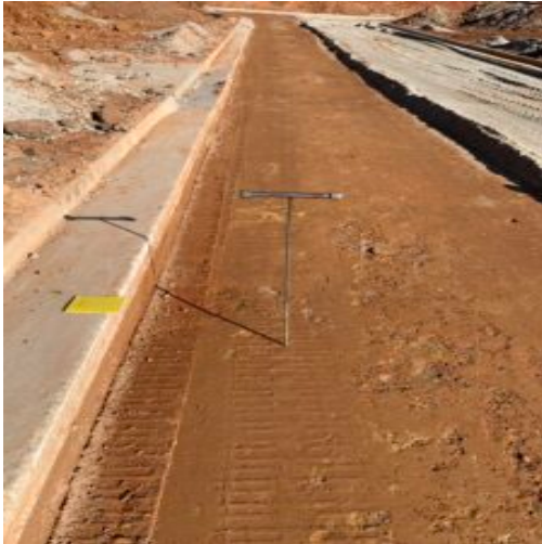
Repaired sub grade observed by probing
