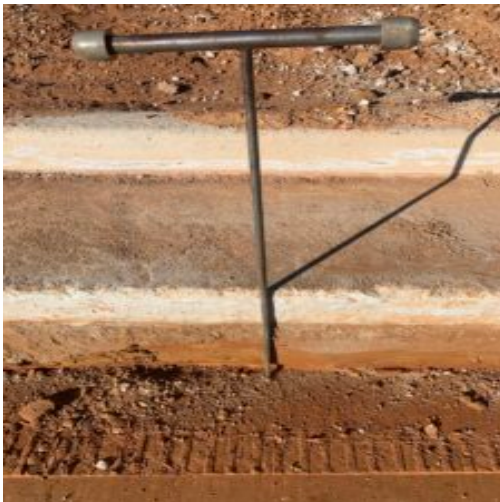
Depth checks ranging from 9" to 14"
