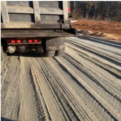
Proof rolling of sub base on Hawthorne having slight to severe movement under traffic. Also in place base stone depths ranging from 3" to six".
