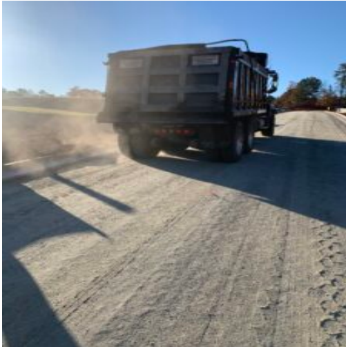
Proof rolling of sub base on Hawthorne having slight to severe movement under traffic. Also in place base stone depths ranging from 3" to six".
