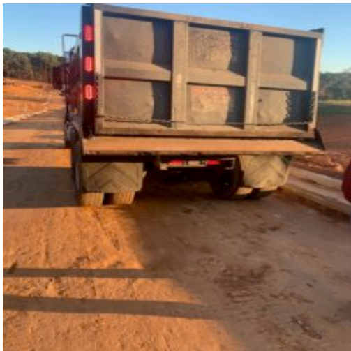
Proof rolling of sub grades at roadway into phase 2
