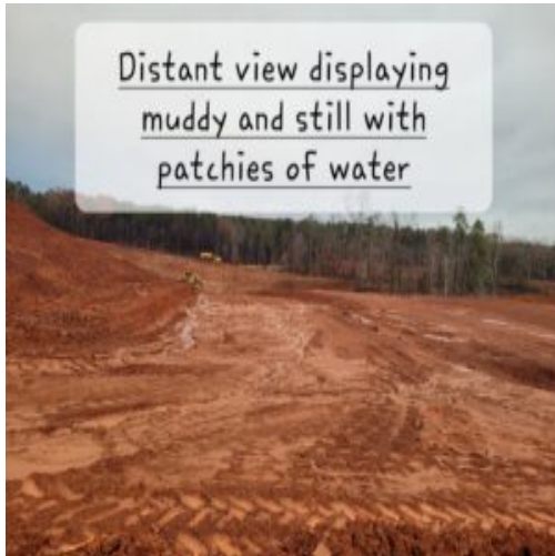
NE view of part of the job site
