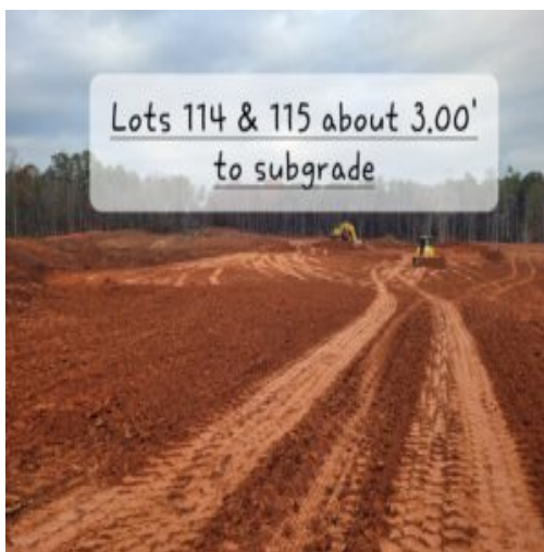
Photo depicting compacted building pads close to sungrade
