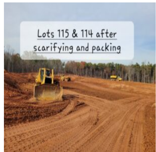
Picture shows lots 114 & 115 scarified and repacked
