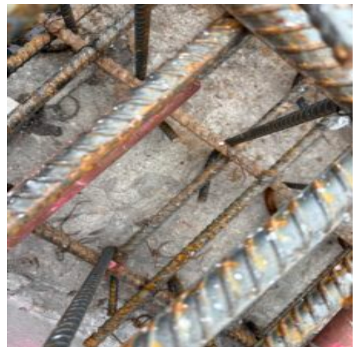
C rebar touching ground
