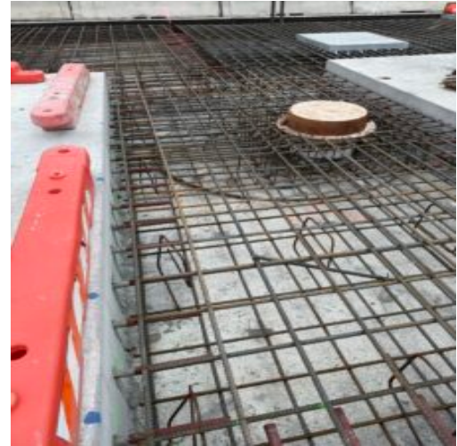
improper clearance
