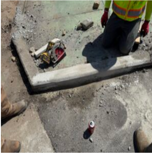
Curb repair area 1
