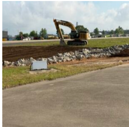
spreading topsoil
