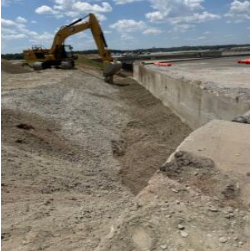
Backfilling
