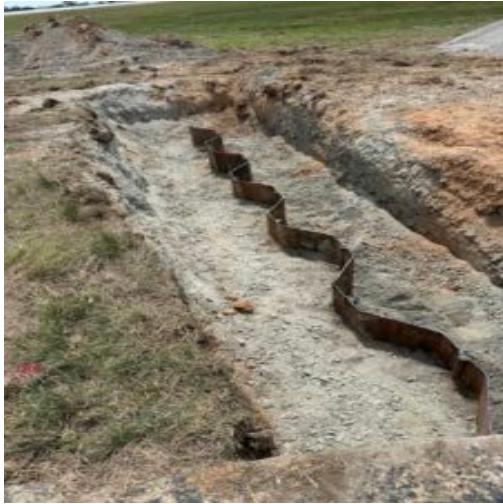
Sheet piles cut below grade
