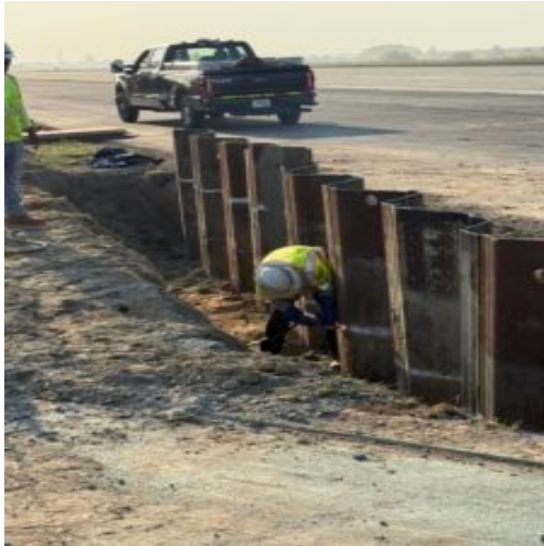
Sheet Piles being cut down
