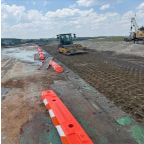
compacting final lift
