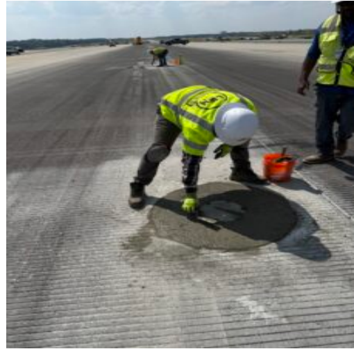
Placing concrete around light cans center runway.
