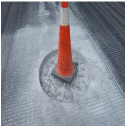
light cans cored before concrete placement
