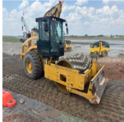
compacting final lift
