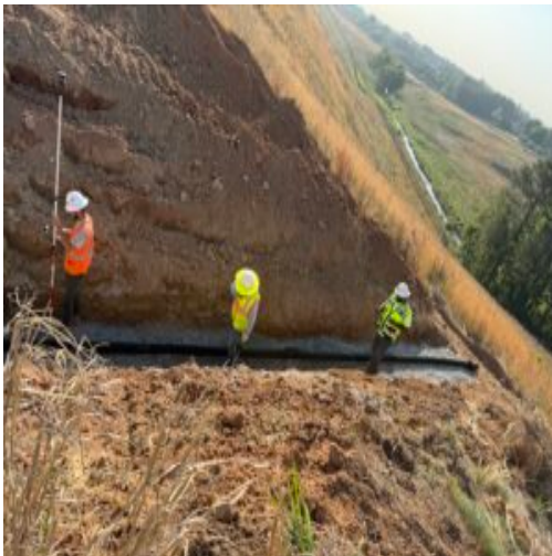
Pipe placement and surveyor verification
