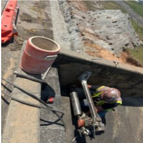
Area 5 Hole drilled through wall for drain
