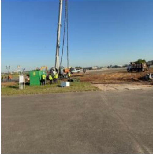
Sheet pile installation
