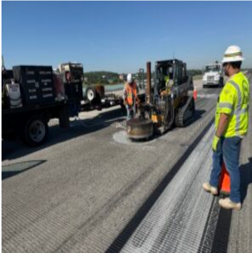
Coring around existing Lights
